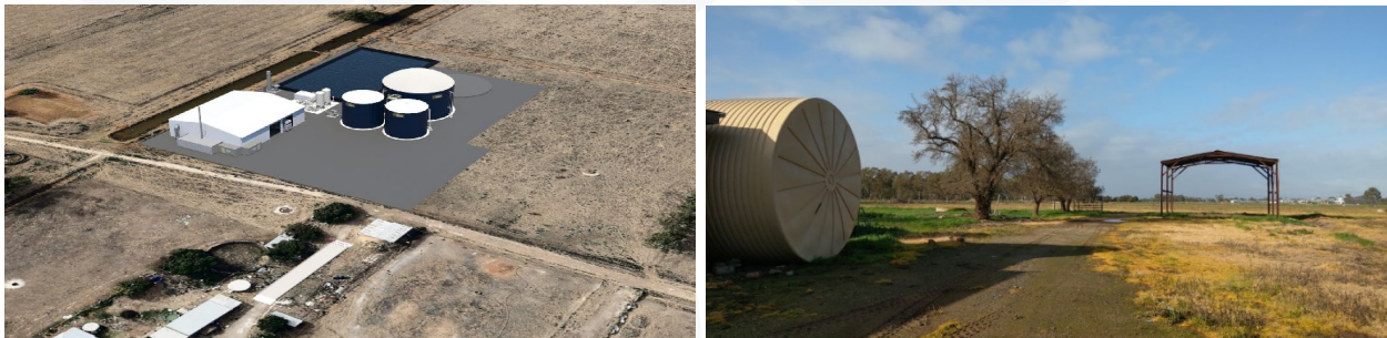
Figure 3.0 & 3.1 DEVO project render and site clearing
