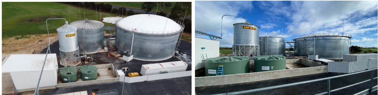
Figure 2.0 & 2.1 Blue Lake Milling nearing completion
