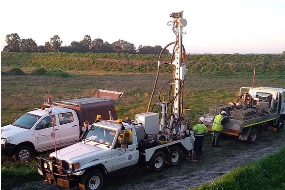
FIGURE 3 : MANTIS 75 DRILL RIG AND SUPPORT TRUCK
