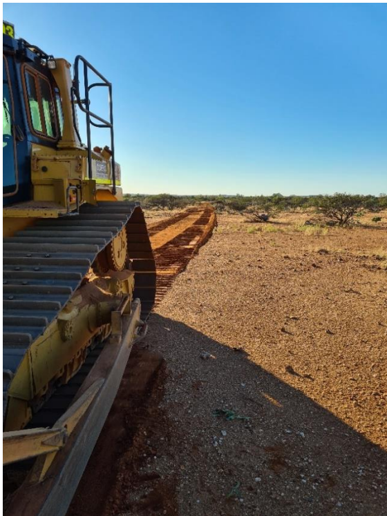
Figure 5: Site access track clearing
