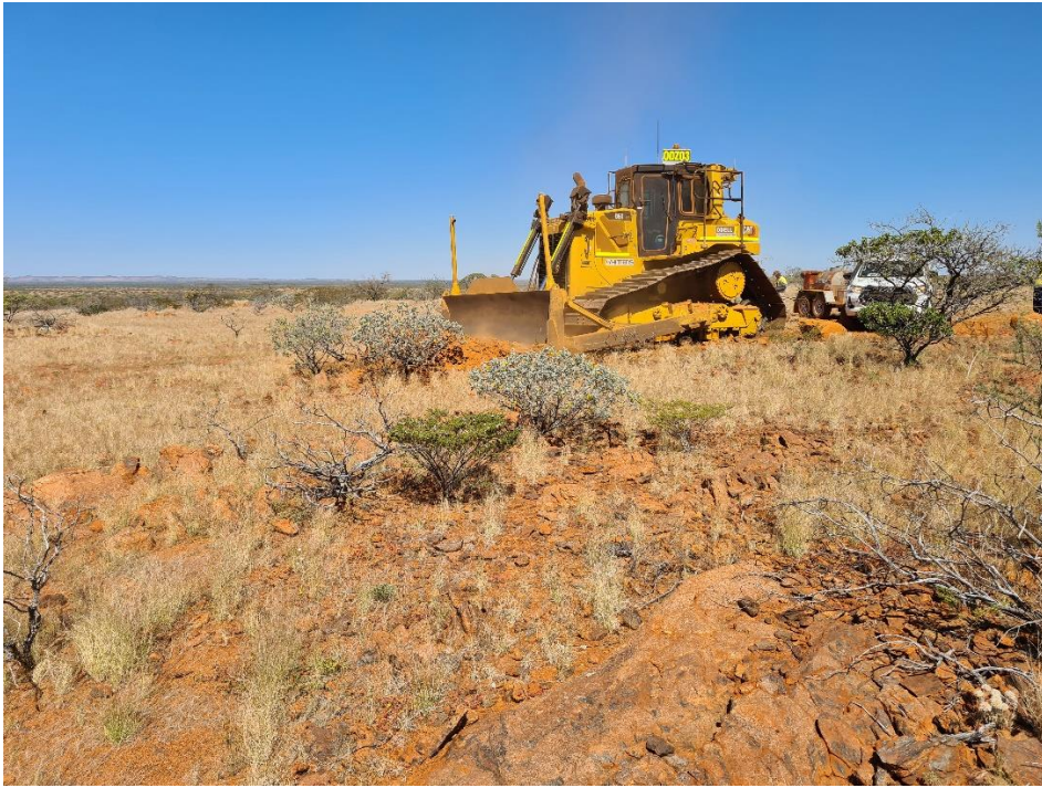
Figure 7: Dozer commencing early works
