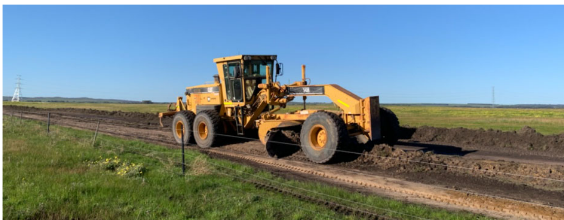
Walyering-5 well pad preparations
