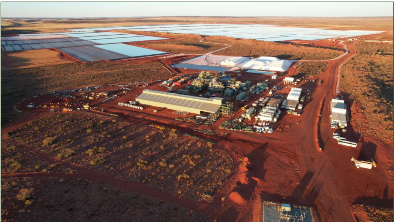
ROM Stockpile and SOP Purification Plant – Viewed from the West
