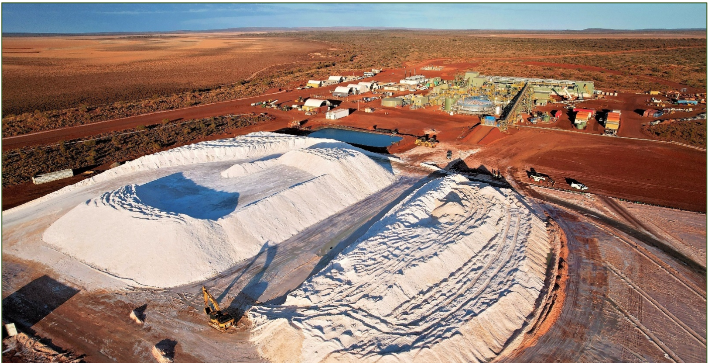
ROM Stockpile and SOP Purification Plant – Viewed from the East
