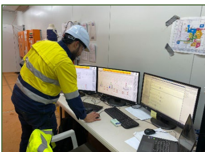
Engineering Control Room
