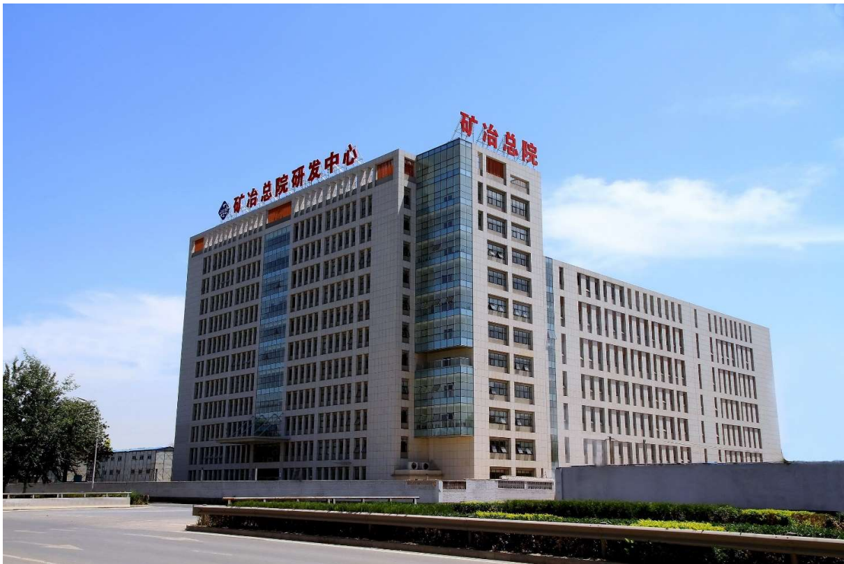
Figure 4: BGRIMM's offices, laboratory facilities, pilot plants are located in Beijing, China
