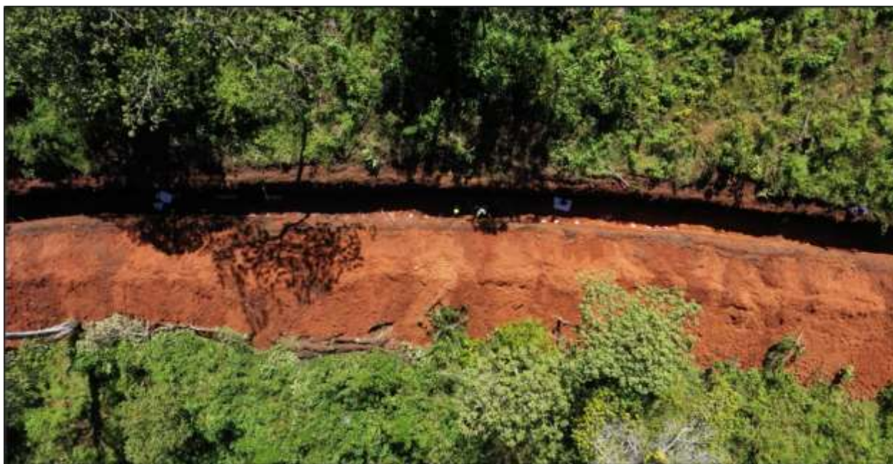
Figure 10 – Megado's team working the first trench at the Babicho Gold Project
