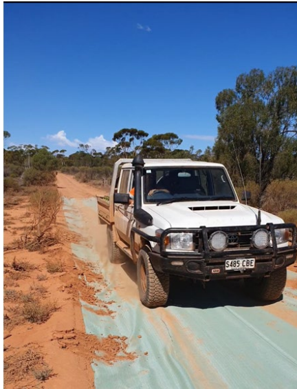
Shade-cloth trialed in 2021 reducing track degradation
