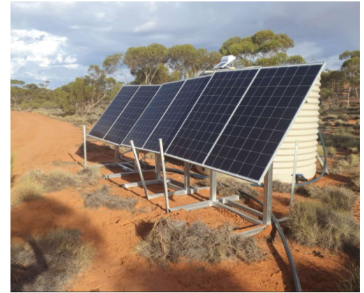
Solar pumping of drilling water up to 25km to reduce environmental impacts
