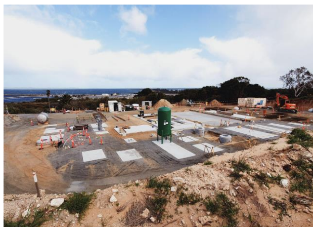
CDP Construction Site at 2 September 2021
