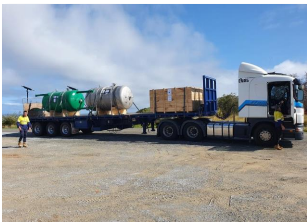
Delivery of equipment for future installation
