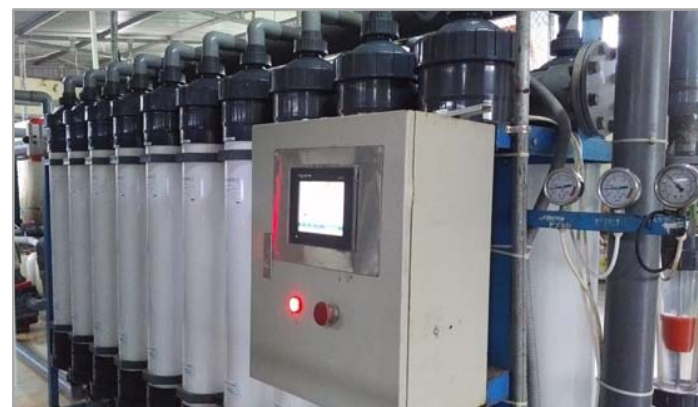
IMAGE: De.mem Ultrafiltration system
