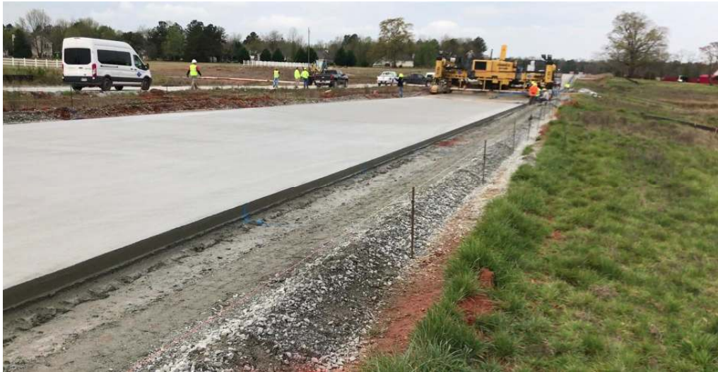
Figure 3. Section of GDOT trial of EdenCrete® in new concrete pavement trial 2017
