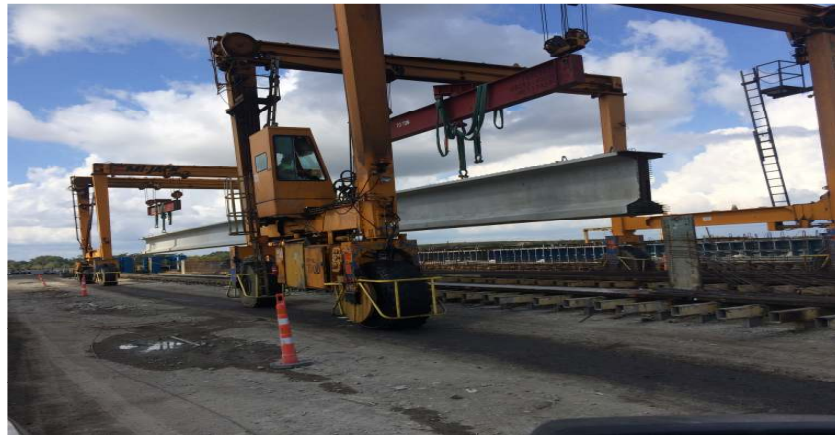
Figure 9. Typical prestressed bridge beam being fabricated
