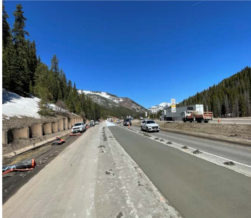
Figure 7. EdenCrete® section of Vail Pass trial being installed
