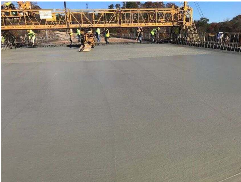
Figure 4. GDOT EdenCrete® bridge trial on bridge over Little River November 2019
