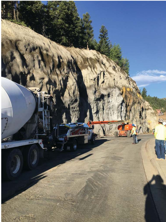
Figure 6. EdenCrete® in use in shotcrete stabilising rock face.
