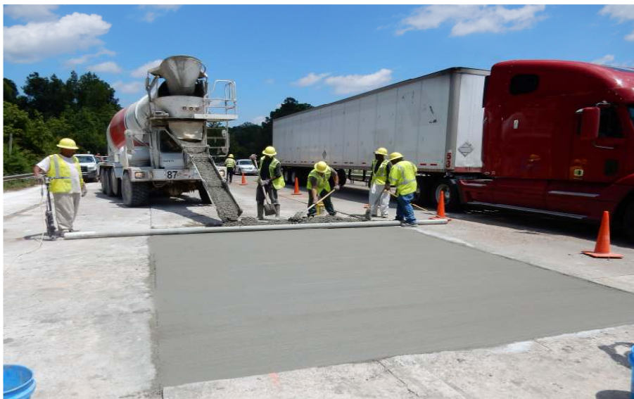
Figure 2. First successful EdenCrete® infrastructure trial - I-20 in Augusta, GA, August 2015
