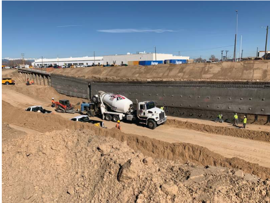
Figure 5. Central 70 – CDOT EdenCrete® Shotcrete project
