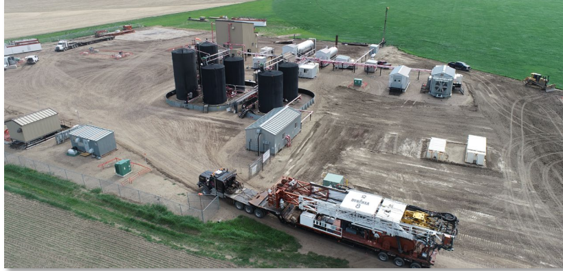
Drilling Rig Move Into 2-29 Battery Site Open Hole Sunburst Drill
