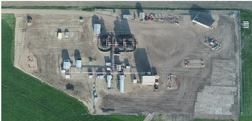
Overhead Drone Shot of the Bantry 2-29 Battery
