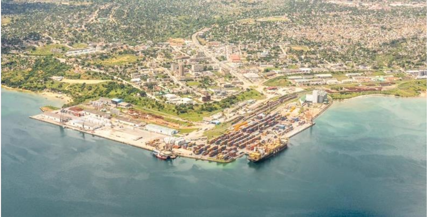
Figure 14: Drone photo looking over the container port at Nacala with loading facilities
