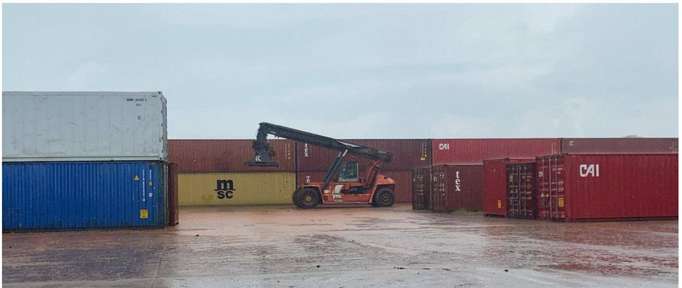
Figure 5: The existing Kanengo rail container terminal connected to the Nacala Logistics Corridor
