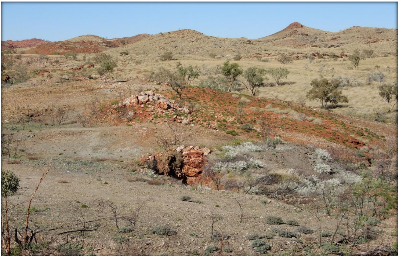
Figure 4: Historic old Shaft over Daltons Shaft No.2 showing the vertical massive quartz lode hosting Gold-Silver and Copper Mineralisation
