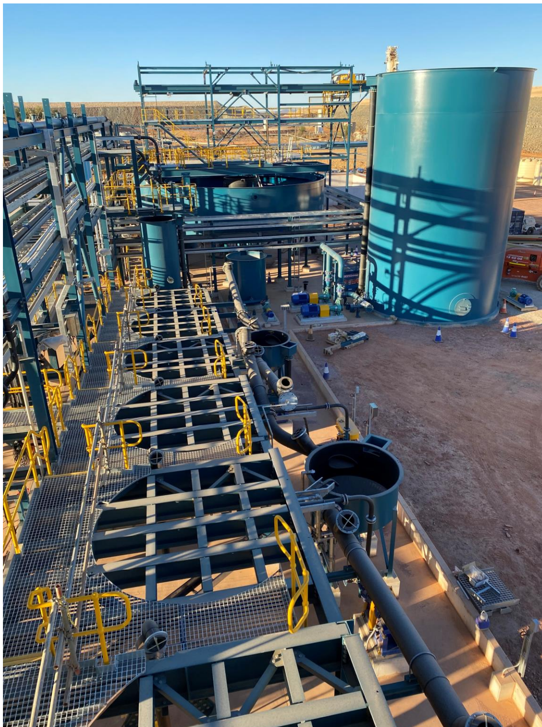
Figure 3: Stage 1 Concentrator construction western side flotation
