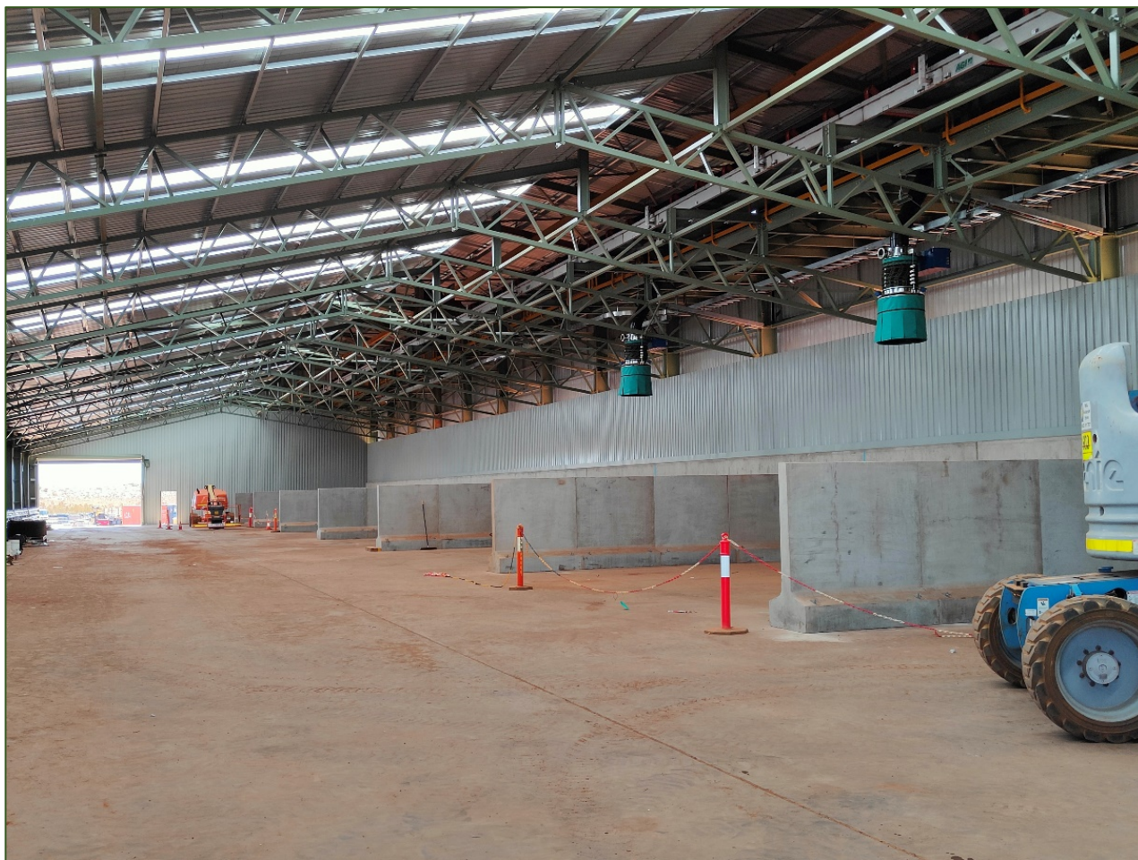
Storage Shed Product Bays with Overhead Delivery Chutes
