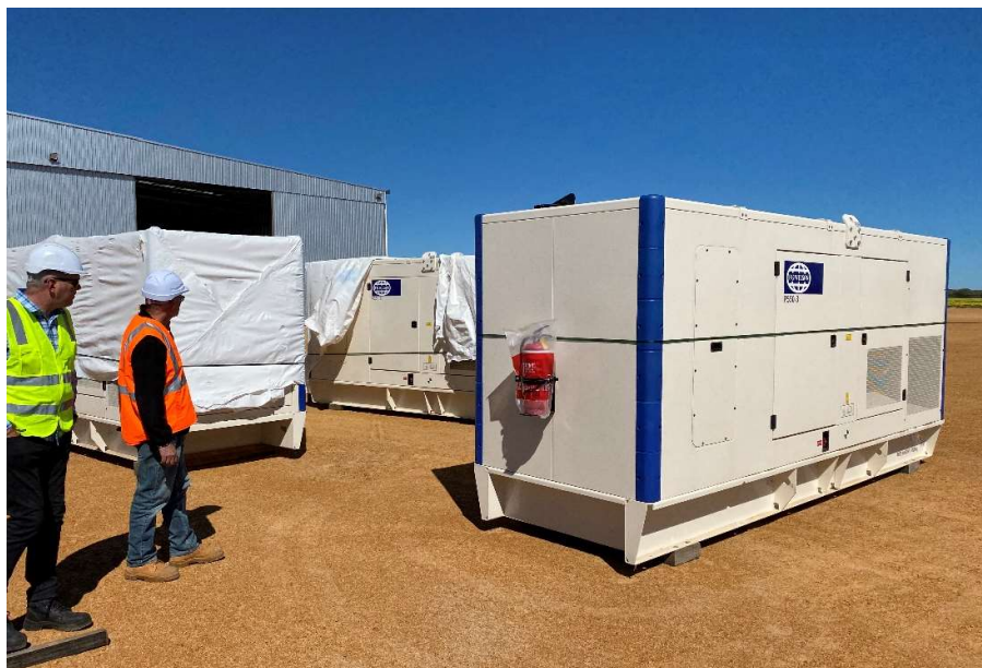
Figure 2. FG Wilson Gensets delivered to the Wickepin Project awaiting installation
