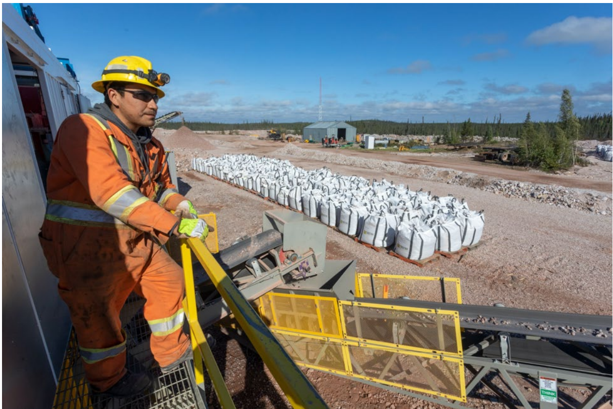
Product staging area at ore sorter reading for relocation to barge lay-down
