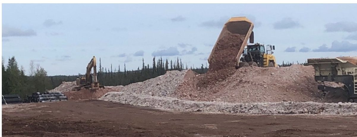
Haul truck placing high-grade ore next to mobile crusher on ROM
