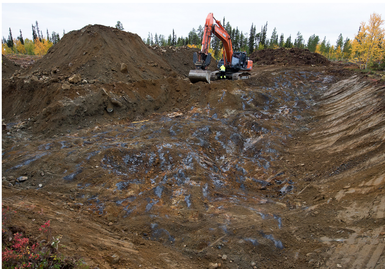
Figure 1 Overburden clearing at trial mine site reveals visible high grade graphite near surface.
