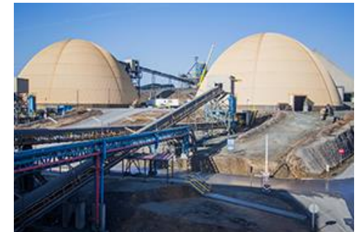
Plant automation with automated SAG mill control, reagent dosing and samples for met accounting
