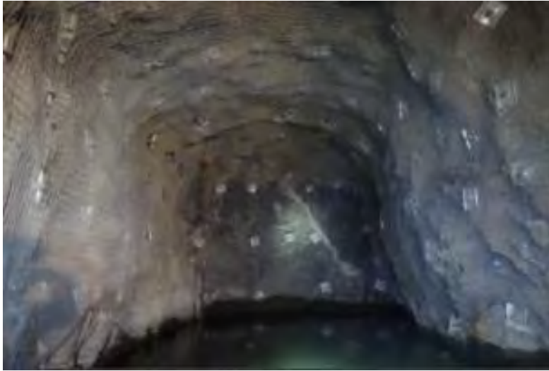
Figure 5-6: Decline face at 1,477 mbs showing high level of reinforcement, including the development face
