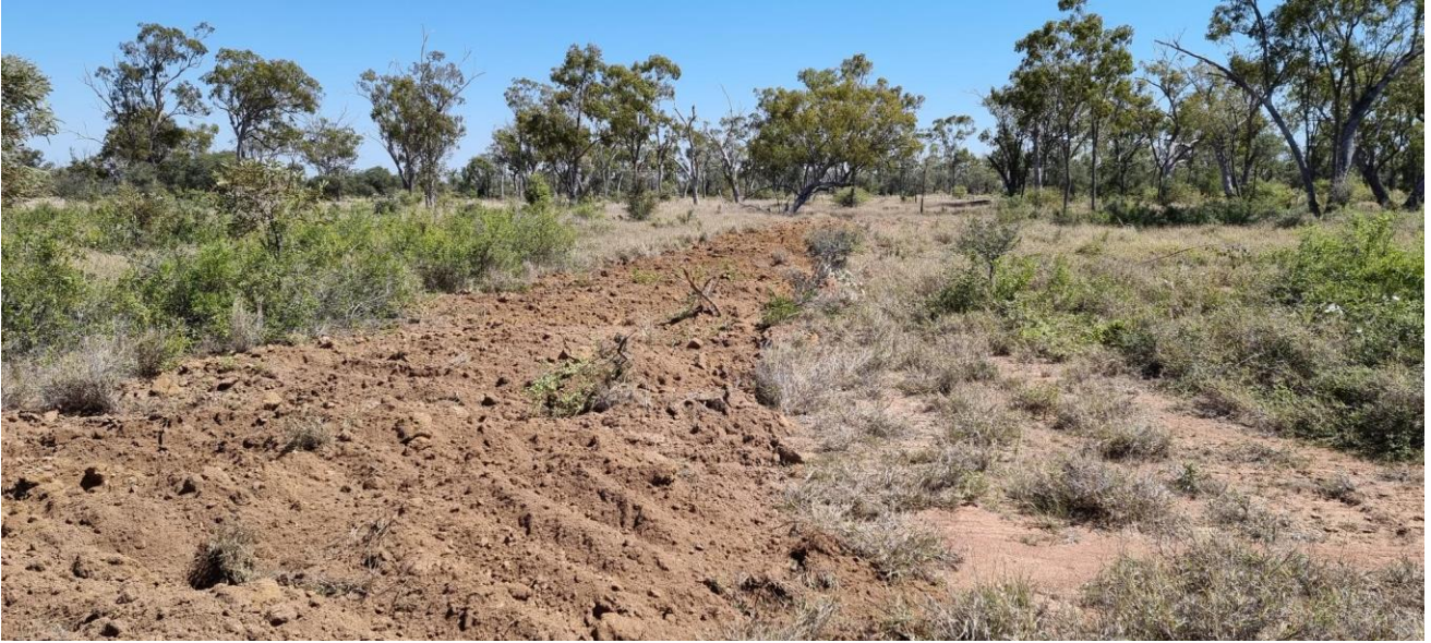
Figure 4. Rehabbed and seeded trench at Red Dog
