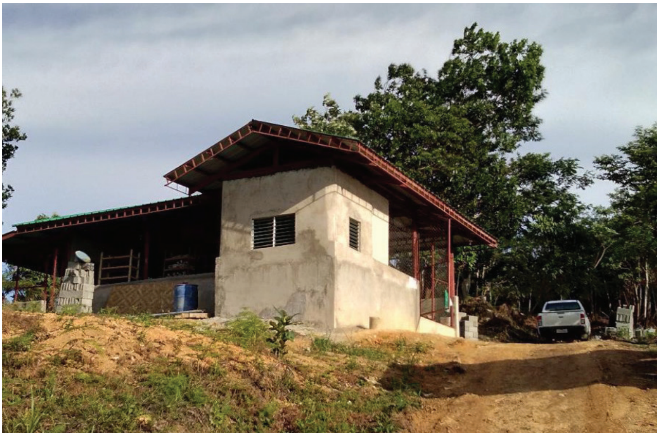
Construction of core shed and accommodation facilities for the exploration team
