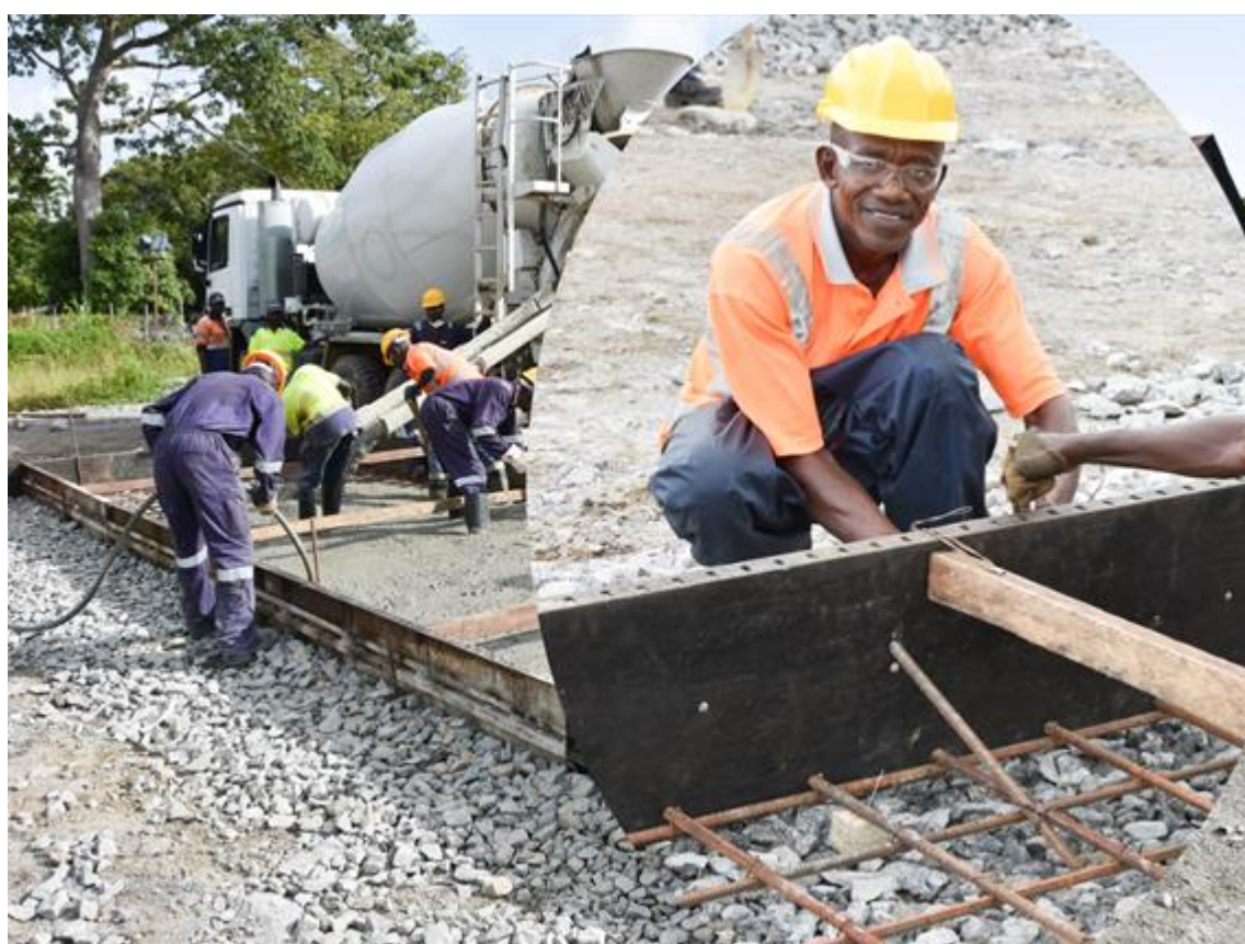
Figure 6: Concrete platforms for the 25 tph plant being poured
