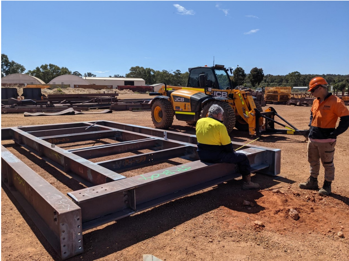
Steel that was part of the Frances Creek Plant, now converted to skid mounts for part of the new Peko Plant.
