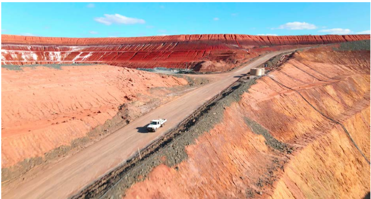
Ramp down to the underground operations at Red October
