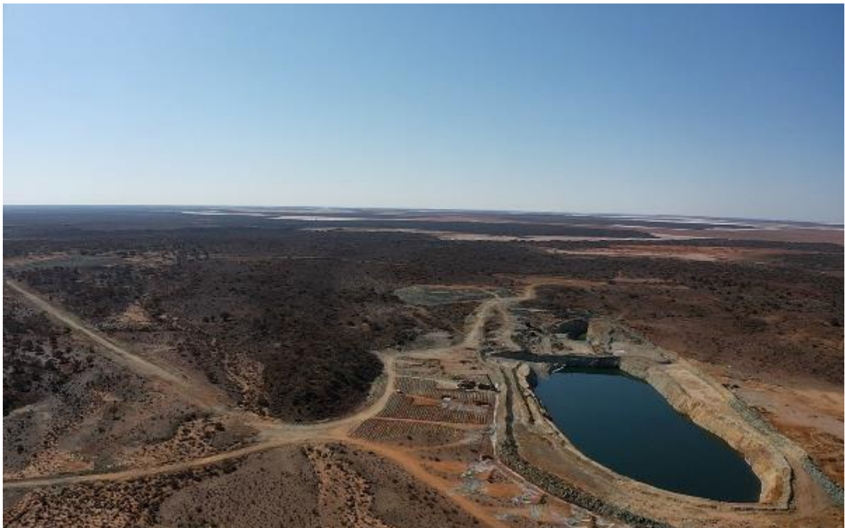
Devon Pit Looking north towards Red October
