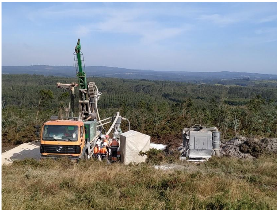
Figure 6 - RC drilling taking place for the emplacement of piezometers
