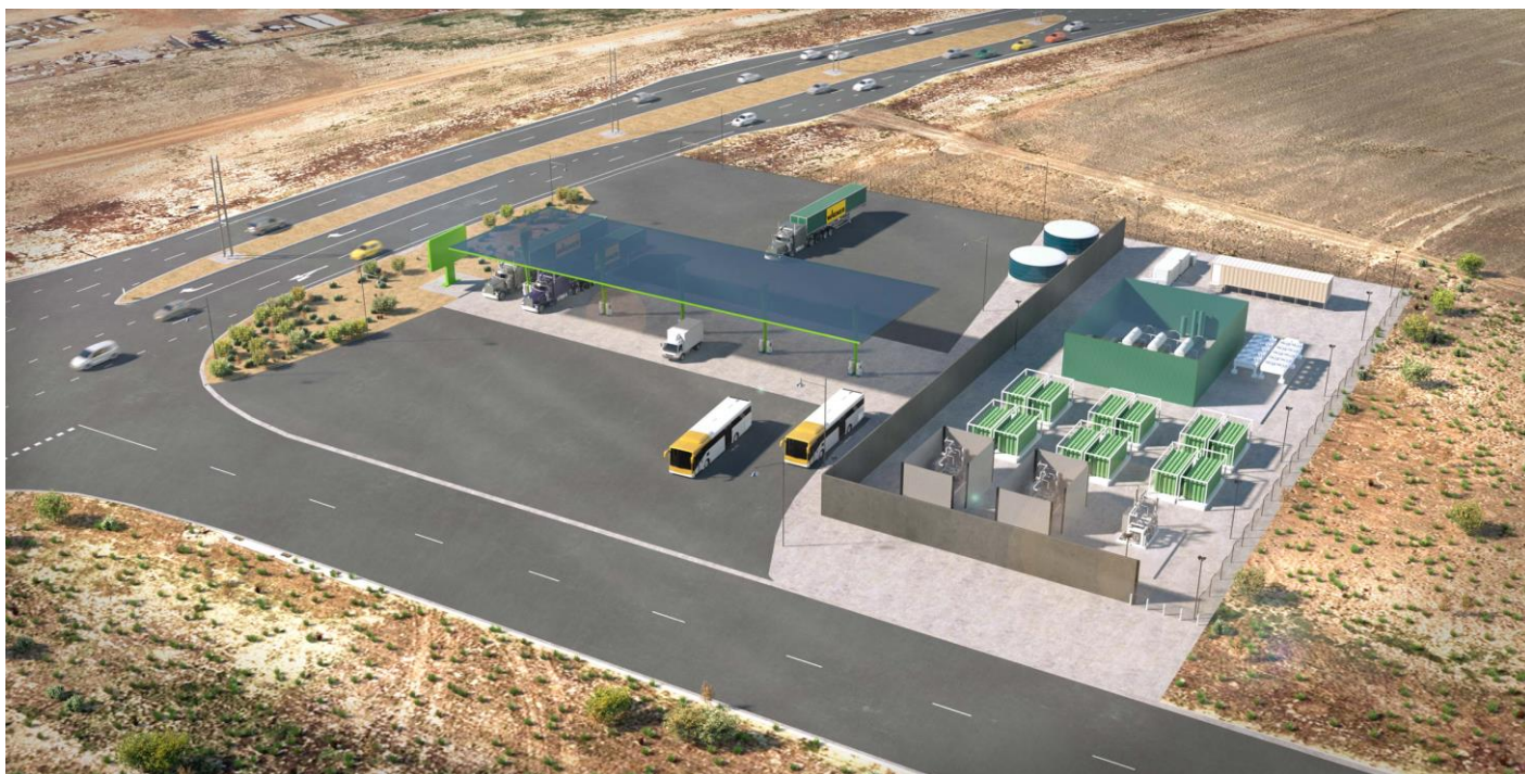
Figure 1: Lion’s initial 2D drawings for a potential 2,000kg/day hydrogen production and refuelling station
