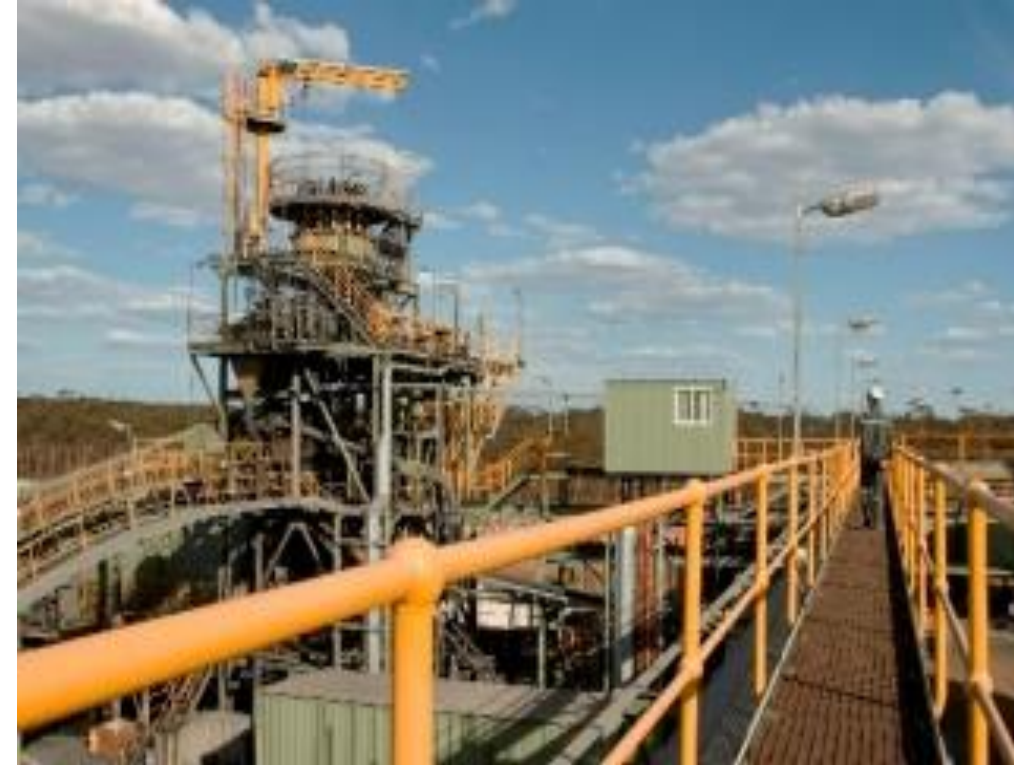
Lake Johnston processing plant
