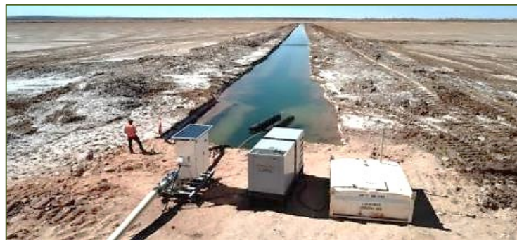
Typical Trench Pump Station
