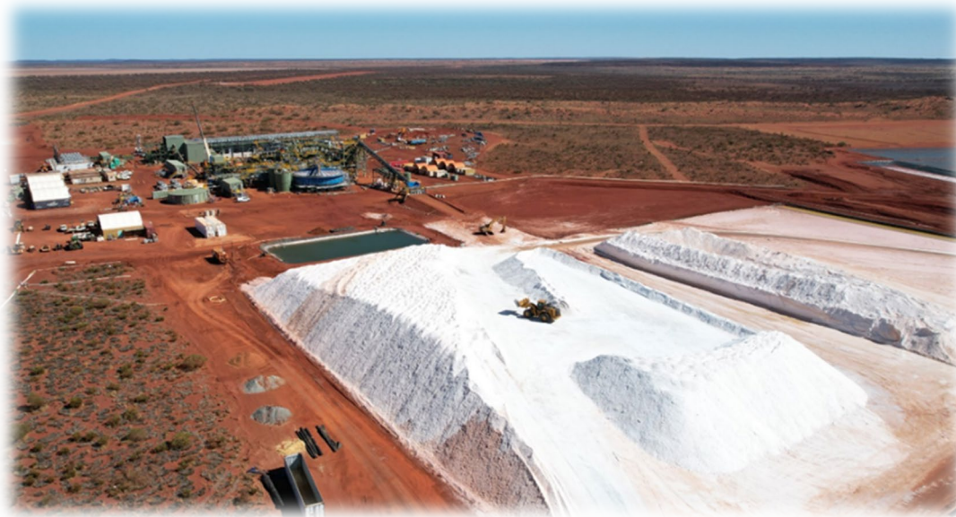
Salt ROM Pad and SOP Purification Plant
