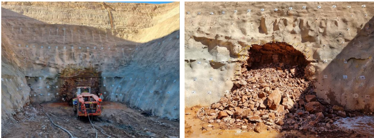
Figure 1 – Jumbo drilling and first cut taken in the Abra Decline
