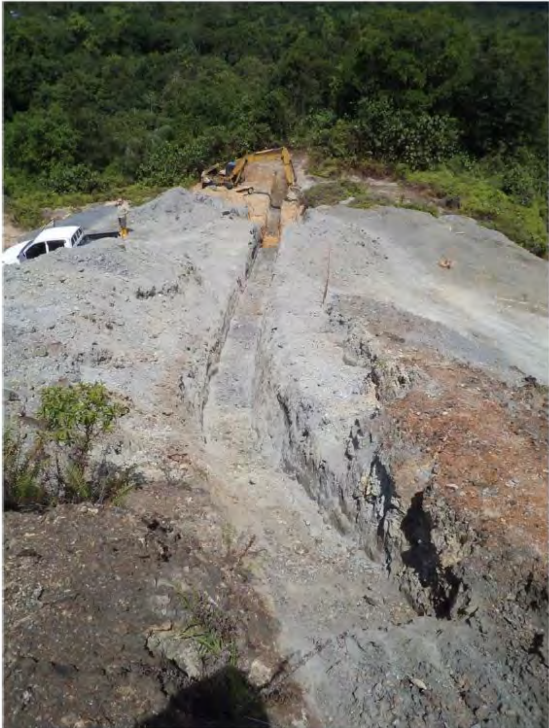
Figure 4-4: Example of Trenching at Jugan Hill
