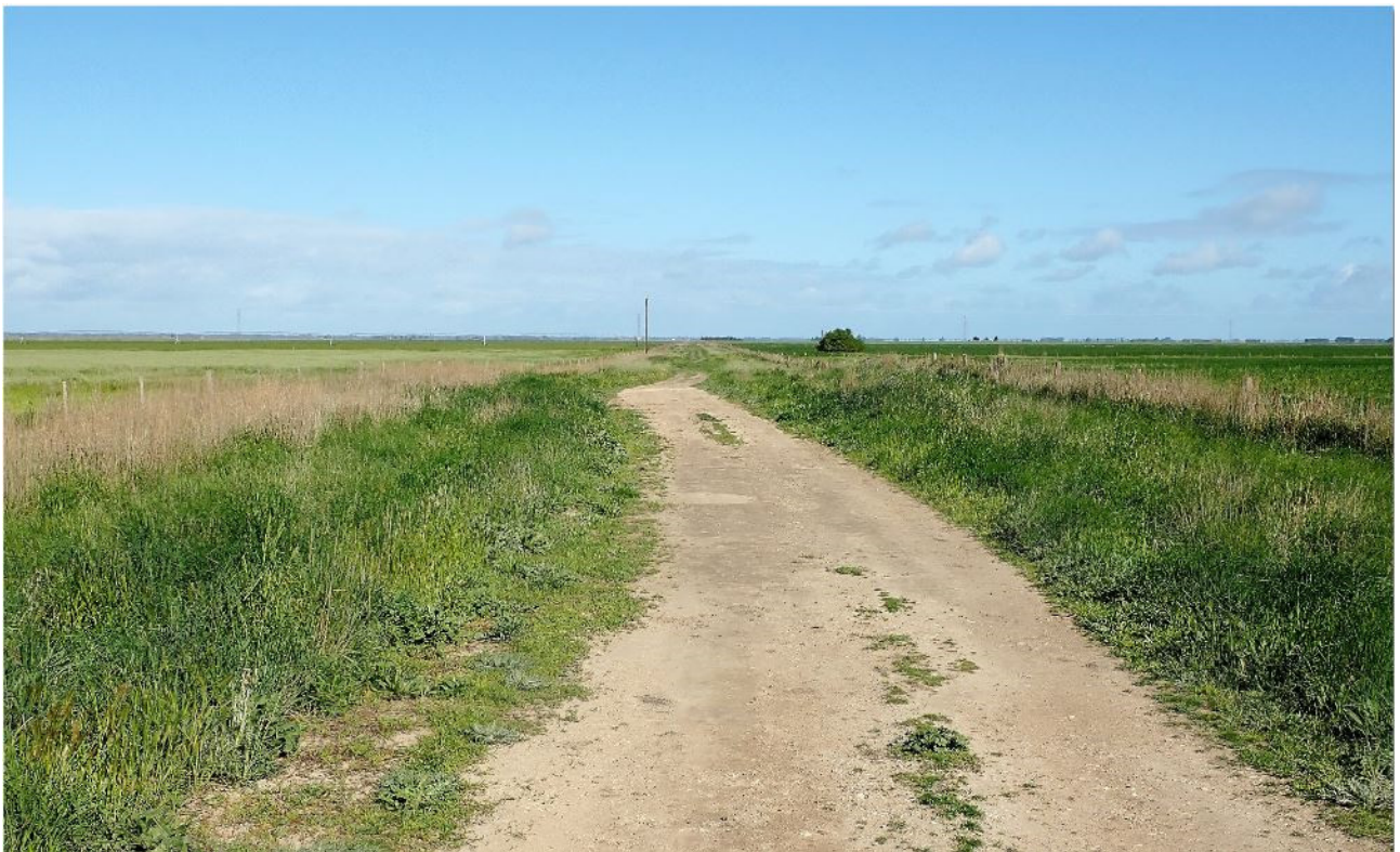
Figure 3: Typical Terrain and Access Road of the Naracoorte Block
