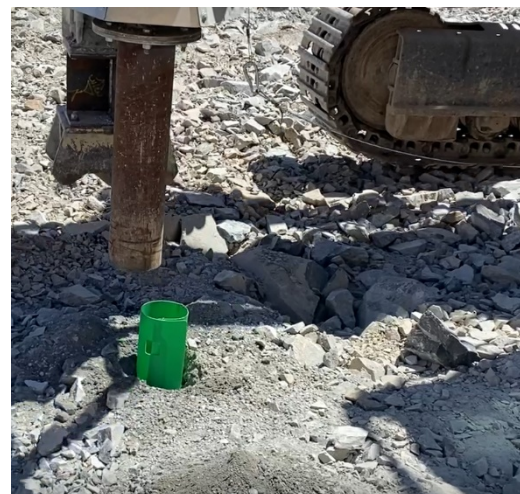
Fig 2. Collar Keeper remains after guide tube removal
