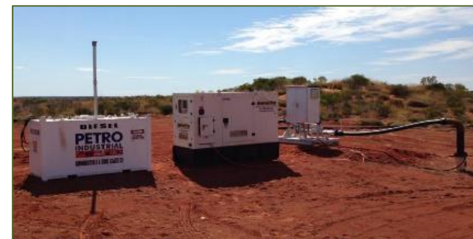
Typical Bore Pump Station
