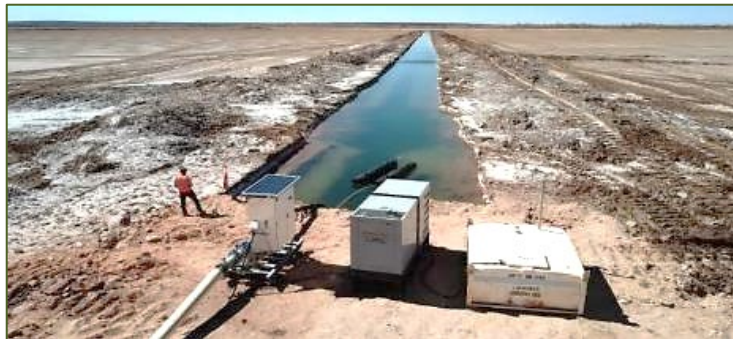
Typical Trench Pump Station
