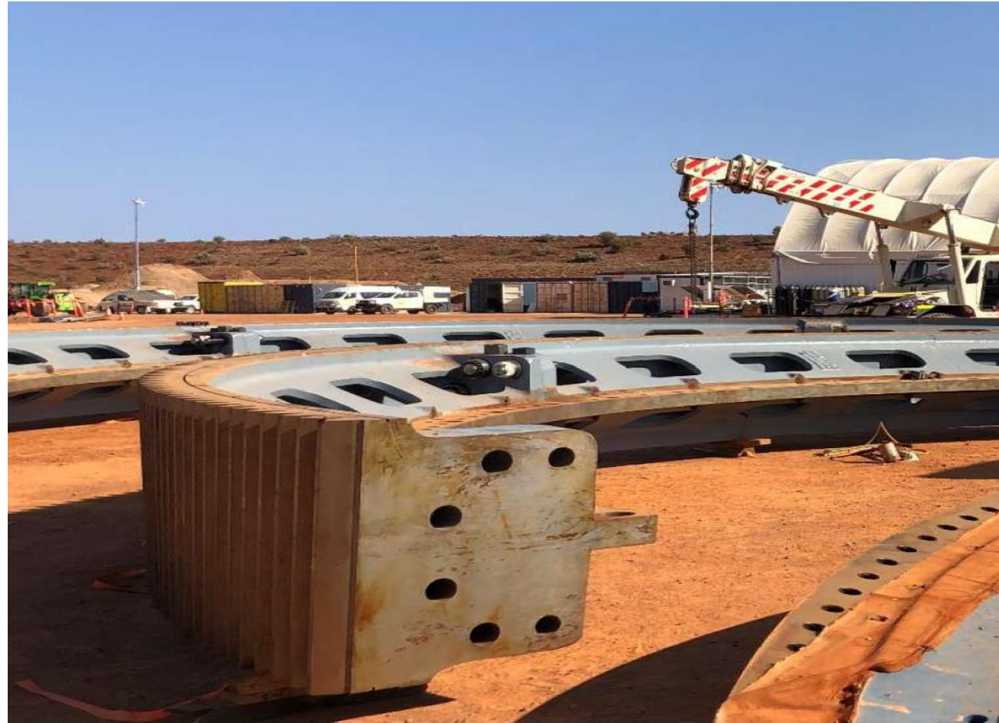
Assembly of girth gear for 36-foot diameter SAG Mill
