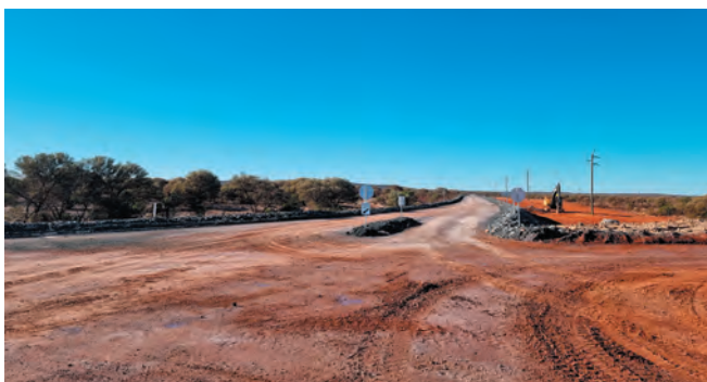
New Cosmos village access road
