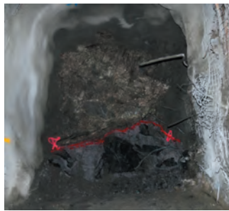
345 S3 south ore drive (4.0m W x 4.5m H) with a face grade of 4.5% Ni
