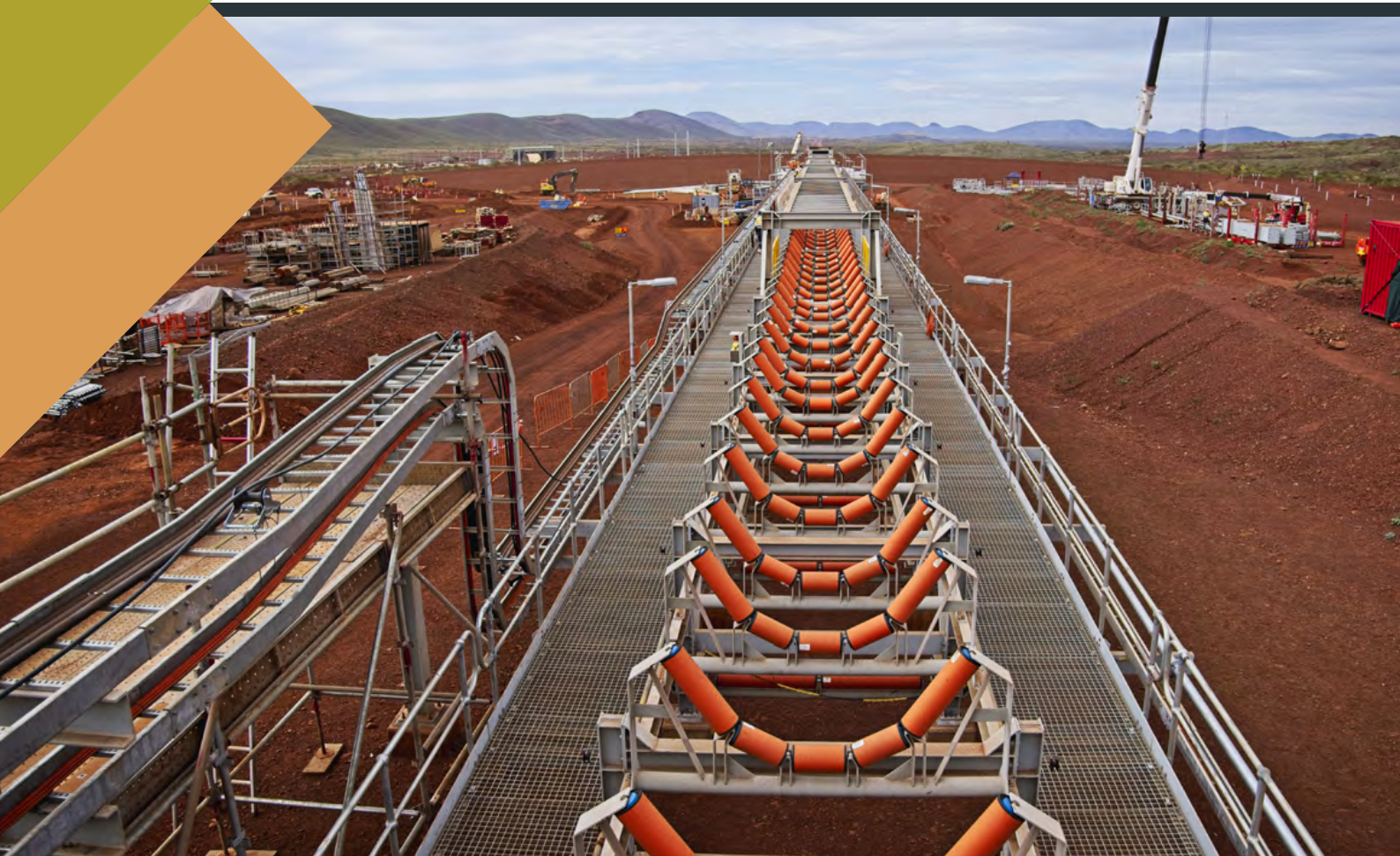
Western Turner Syncline Phase 2 Project, Western Australia
