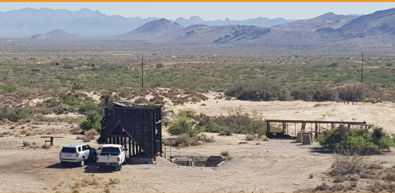
Shaft, ore bin, plant site & tailings at Arizona-Magma (Diana) Mine
