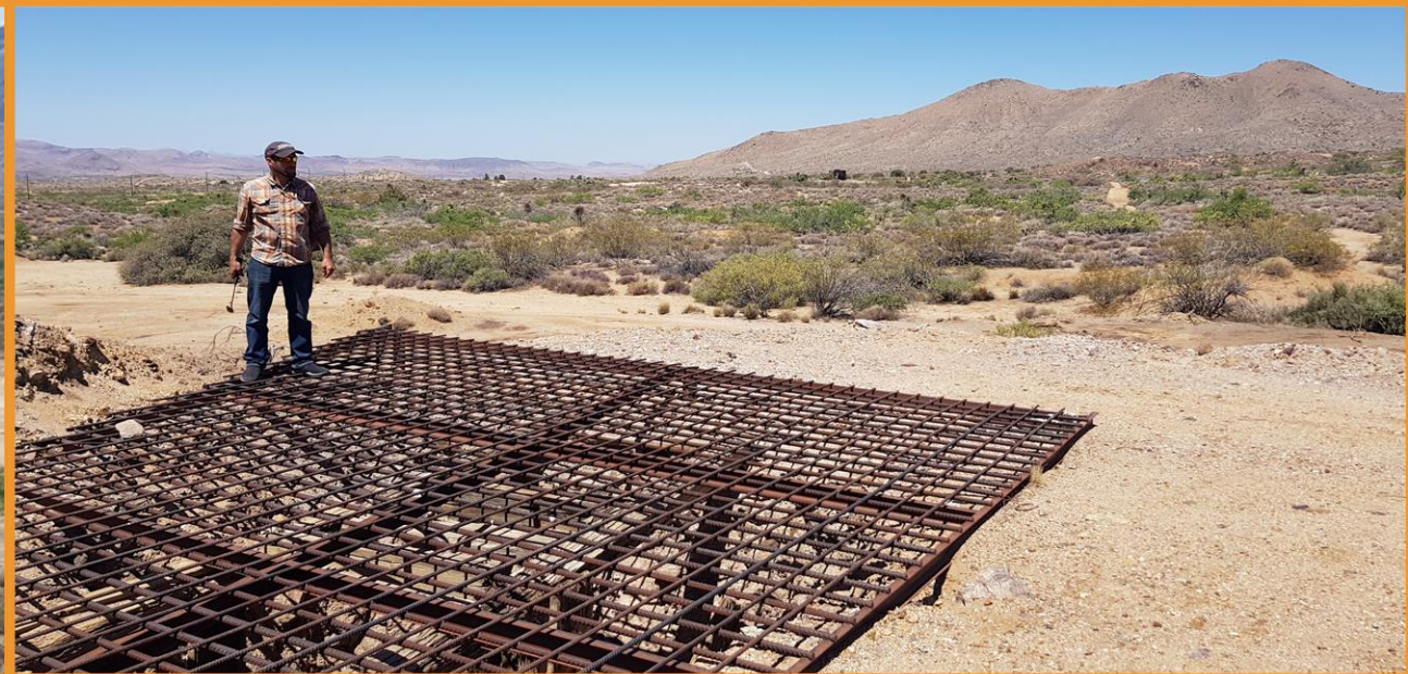
Merrimac Mine Shaft
