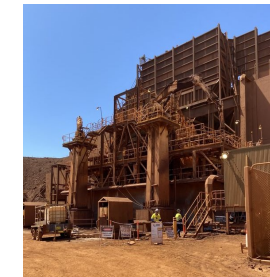
FMG Scope: Jaw Crusher Shutdown – Cloud Break
