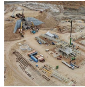
FIRST QUANTUM MINERALS Scope: Structural/Mechanical and Electrical/Instrumentation Installation
