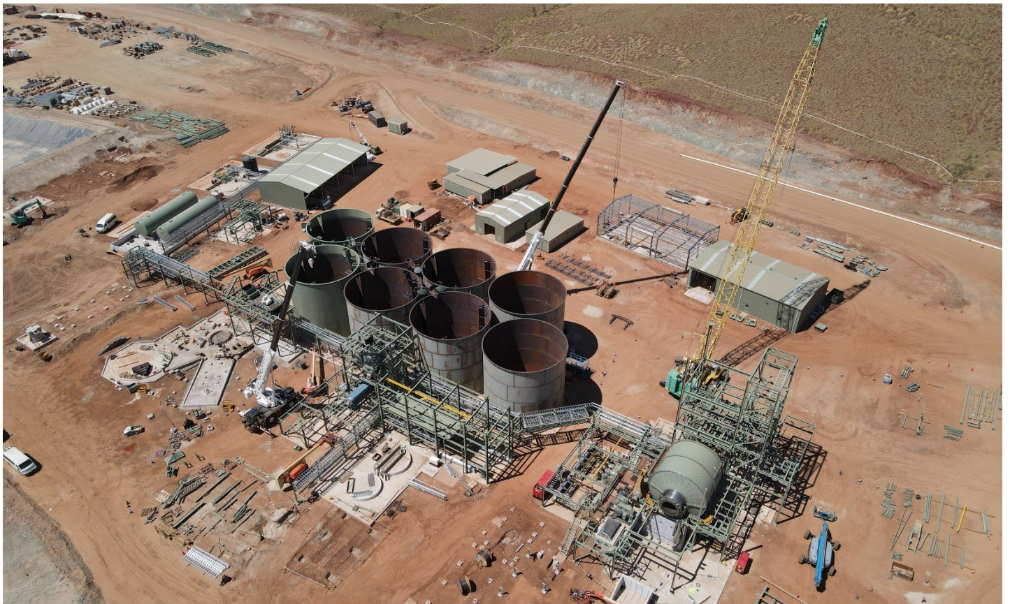
Figure 2: Mill and CIL tank area
