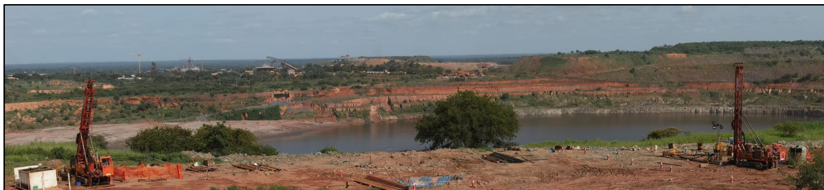
Drilling in progress at Morila NW
