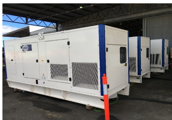
Figure 3. Factory Acceptance Testing at AllightSykes’ Landsdale location
