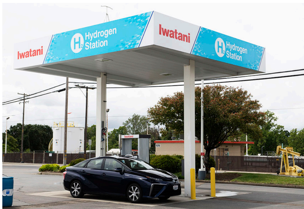
Image 2: Example of hydrogen refuelling station in Sacramento, California.
