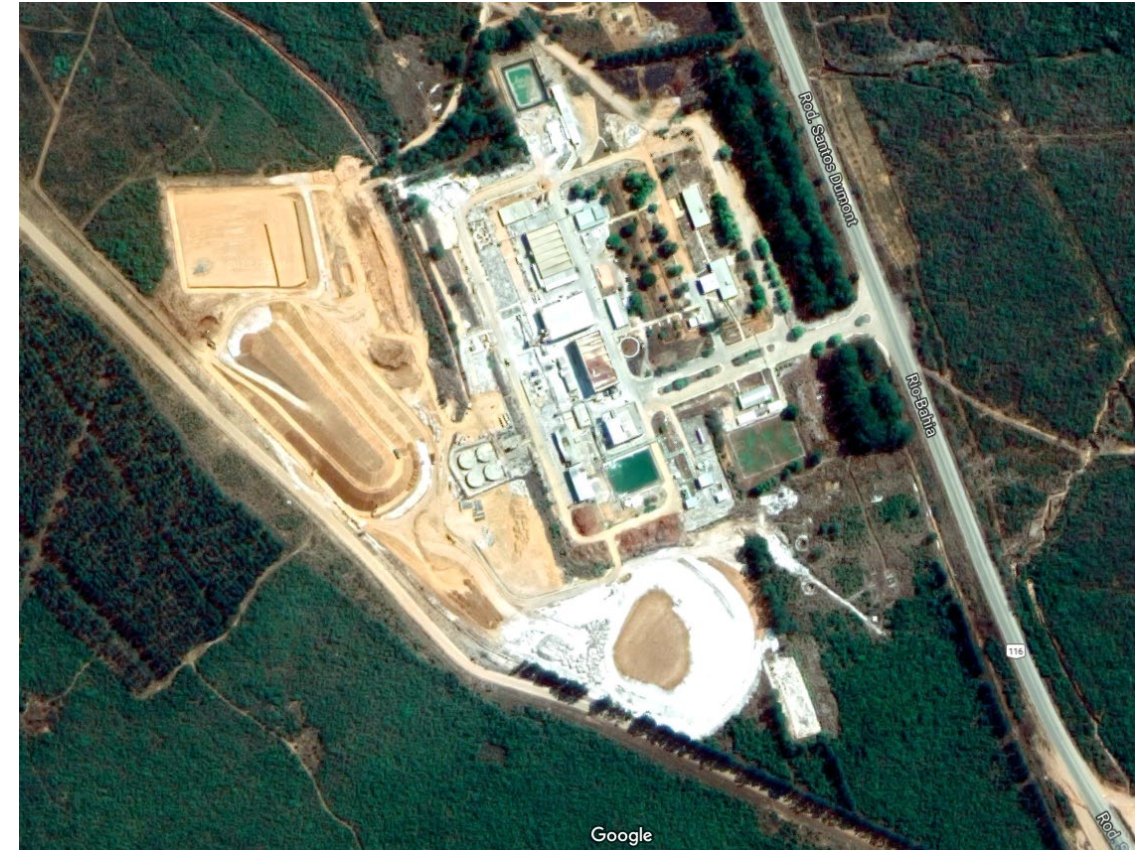
Divisa Alegre Lithium Hydroxide Plant Mina Gerais, Brazil 140km from LRS Pegmatites
