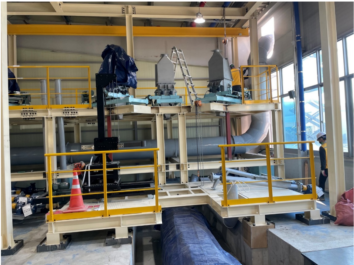
Figure 3 - Installation of Neodymium Furnace Infrastructure
