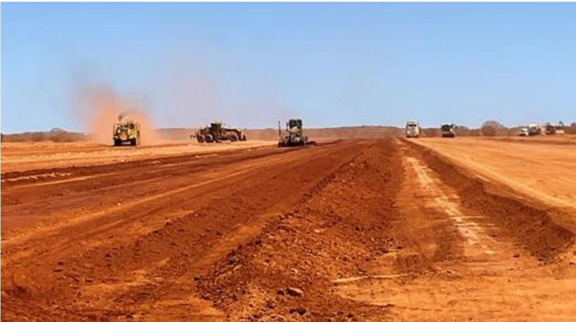
*Figure 2. Foundation works for airstrip (photograph date 10<sup>th</sup> October 2021).*
