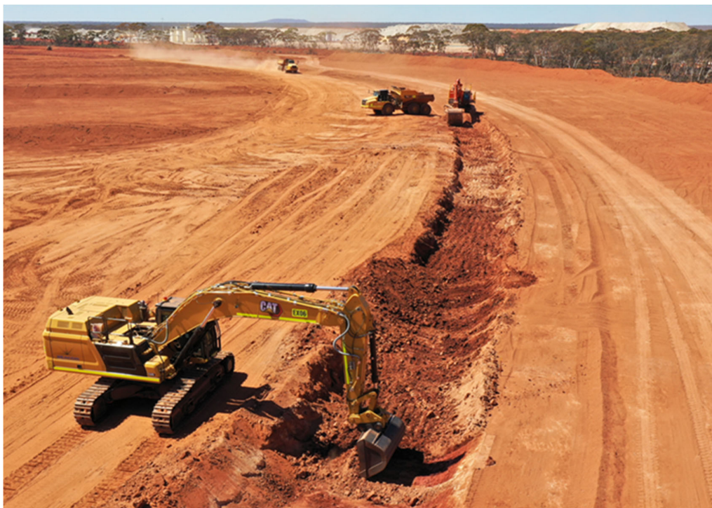
Figure 2: Excavators preparing cut off trench beneath Jaurdi TSF
