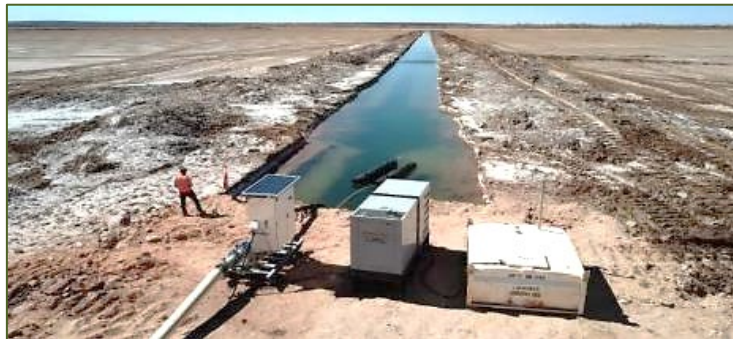
Typical Trench Pump Station
