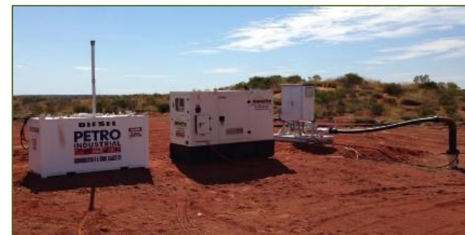
Typical Bore Pump Station
