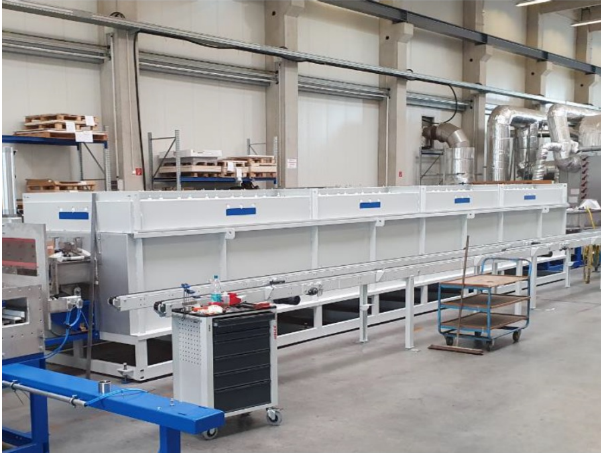
Talga EVA anode coating oven under construction
